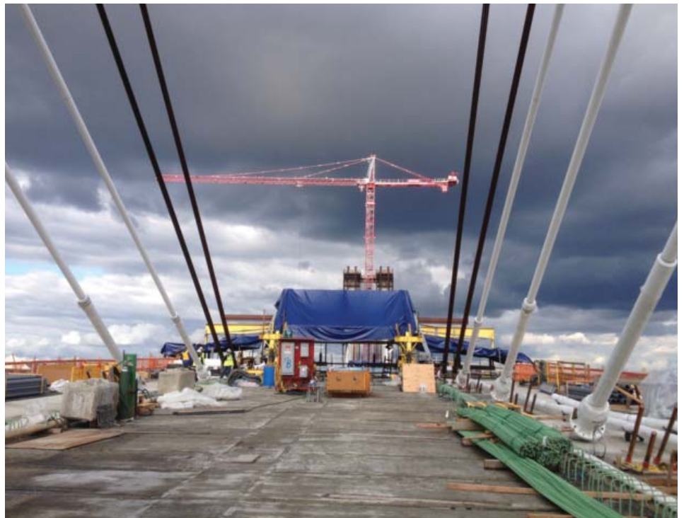
Willamette River Bridge, courtesy of Tyler Street.
