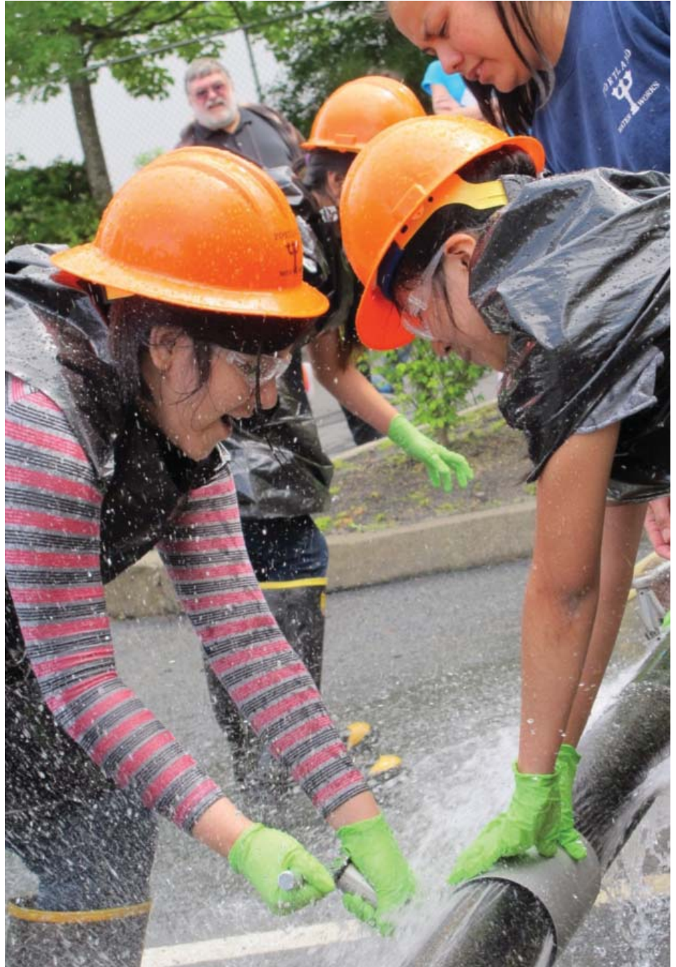
High school girls fix a water main break in the Portland Water Bureau’s workshop. The 2014 Women in Trades Career Fair will be held May 8-10 at the NECA-IBEW Electrical Training Center, 16021 N.E. Airport Way, Portland. For more information about the event or how to register your school, visit www.tradeswomen.net/fair .
