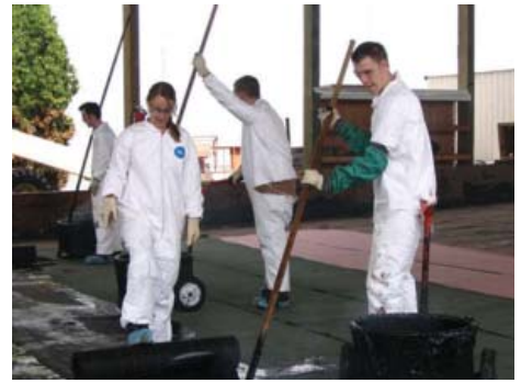
Laying tar at the Roofers.
